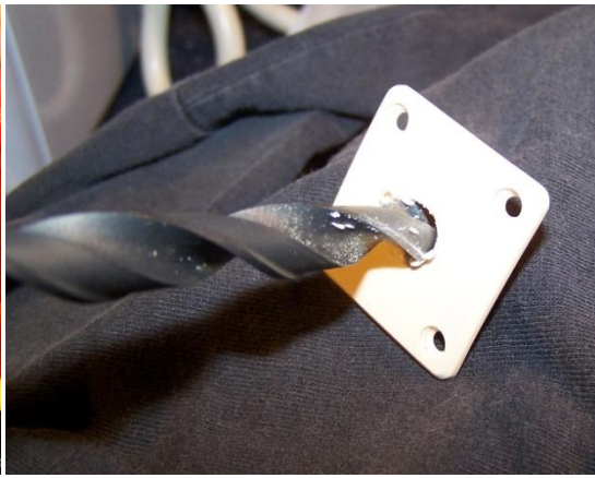
Fig. 13 Open up the jack plate so that the new jack will fit through it.
